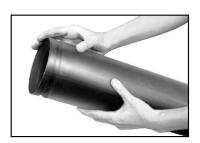
1. INSPECT PIPE ENDS: For optimum sealing by the gasket, the exterior surface of the pipe ends must be free from any indentations, projections, roll marks or other harmful surface defects such as loose paint, scale, dirt, chips, grease and rust.
